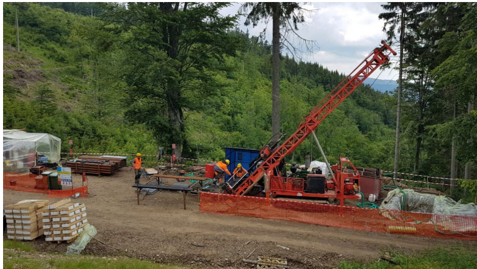
Figure 1: Drilling underway on first hole KBDD-001 at Kolba.
