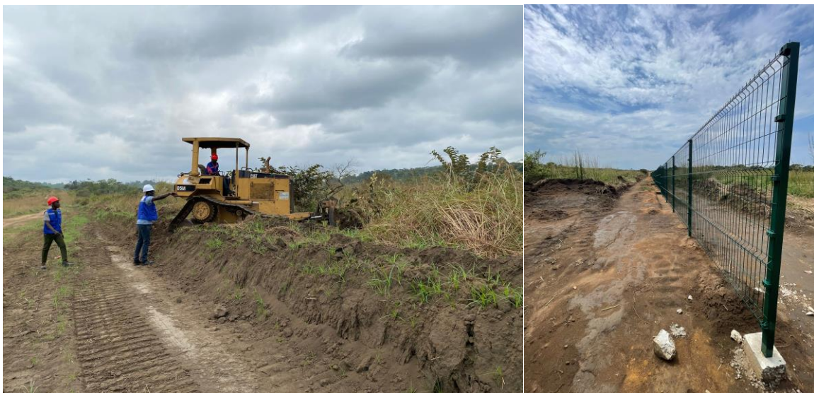
Figure 1 – Subantando Site Clearing and Fencing anticipated to be completed by 9 June 2023.
