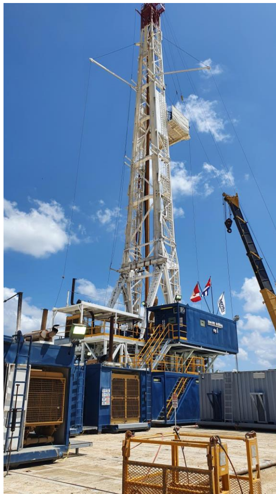
Figure 1 - Drilling rig installation nearing completion
