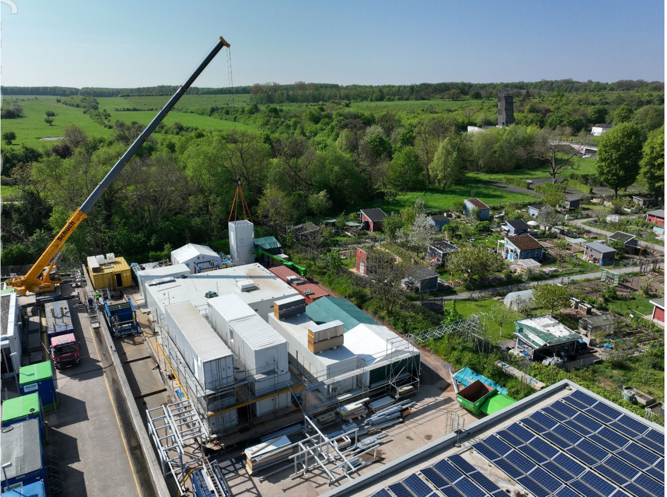
Figure 1: Vulcan's LEOP Plant, under construction
