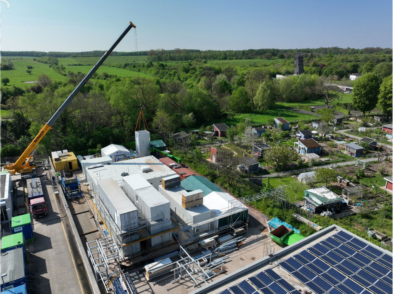
Figure 1: Vulcan's LEOP Plant, under construction
