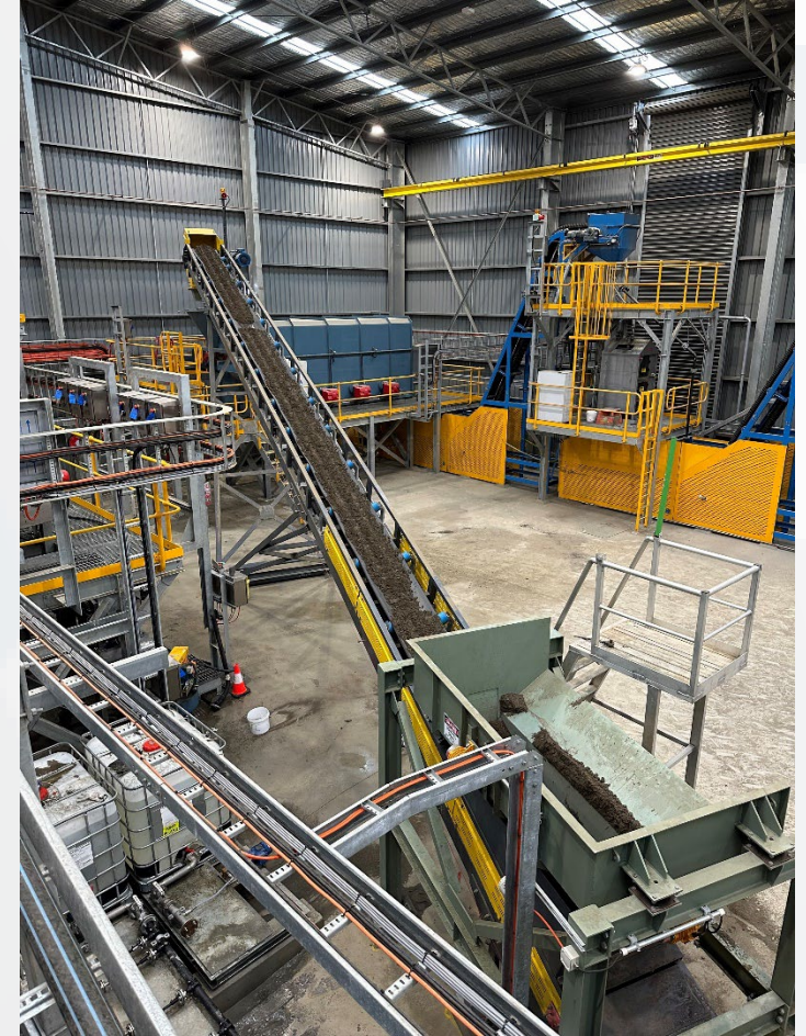
Concentrate Dryer and Magnetic Separator
