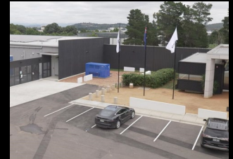
Intellicentre 5 South Bunker, Canberra
