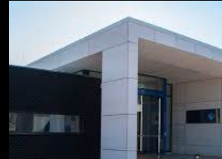
Intellicentre 4 Bunker, Canberra
