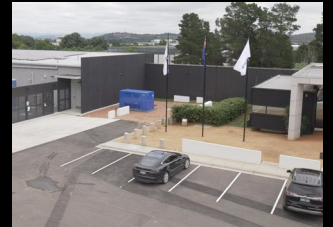
Intellicentre 5 South Bunker, Canberra
