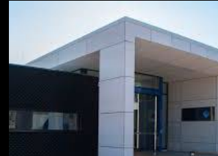
Intellicentre 4 Bunker, Canberra
