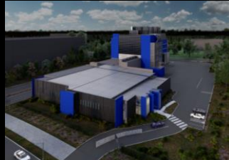
Intellicentre 3 East Macquarie Park
