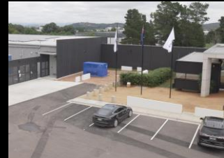
Intellicentre 5 South Bunker, Canberra
