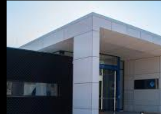
Intellicentre 4 Bunker, Canberra
