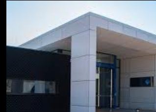
Intellicentre 4 Bunker, Canberra
