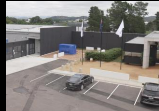
Intellicentre 5 South Bunker, Canberra
