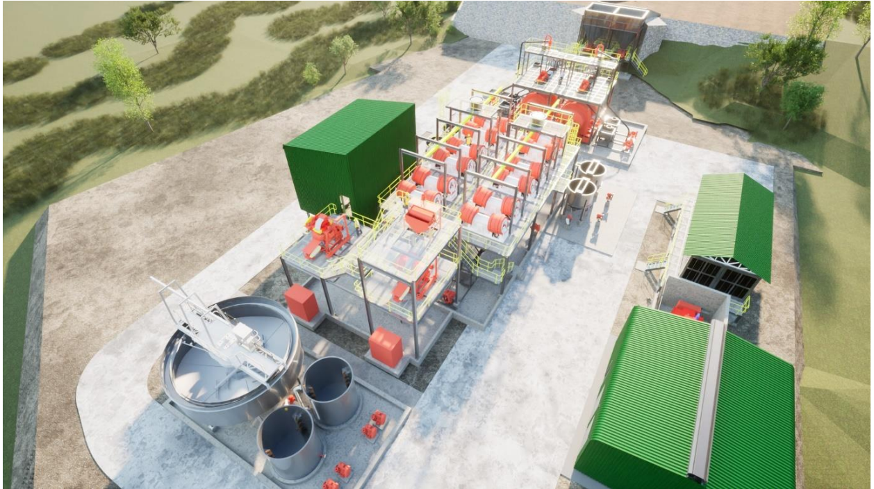
Image 3: Elevated view of the recovery circuit and tailings thickener.
