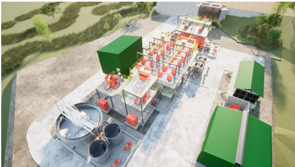
Image 3: Elevated view of the recovery circuit and tailings thickener.
