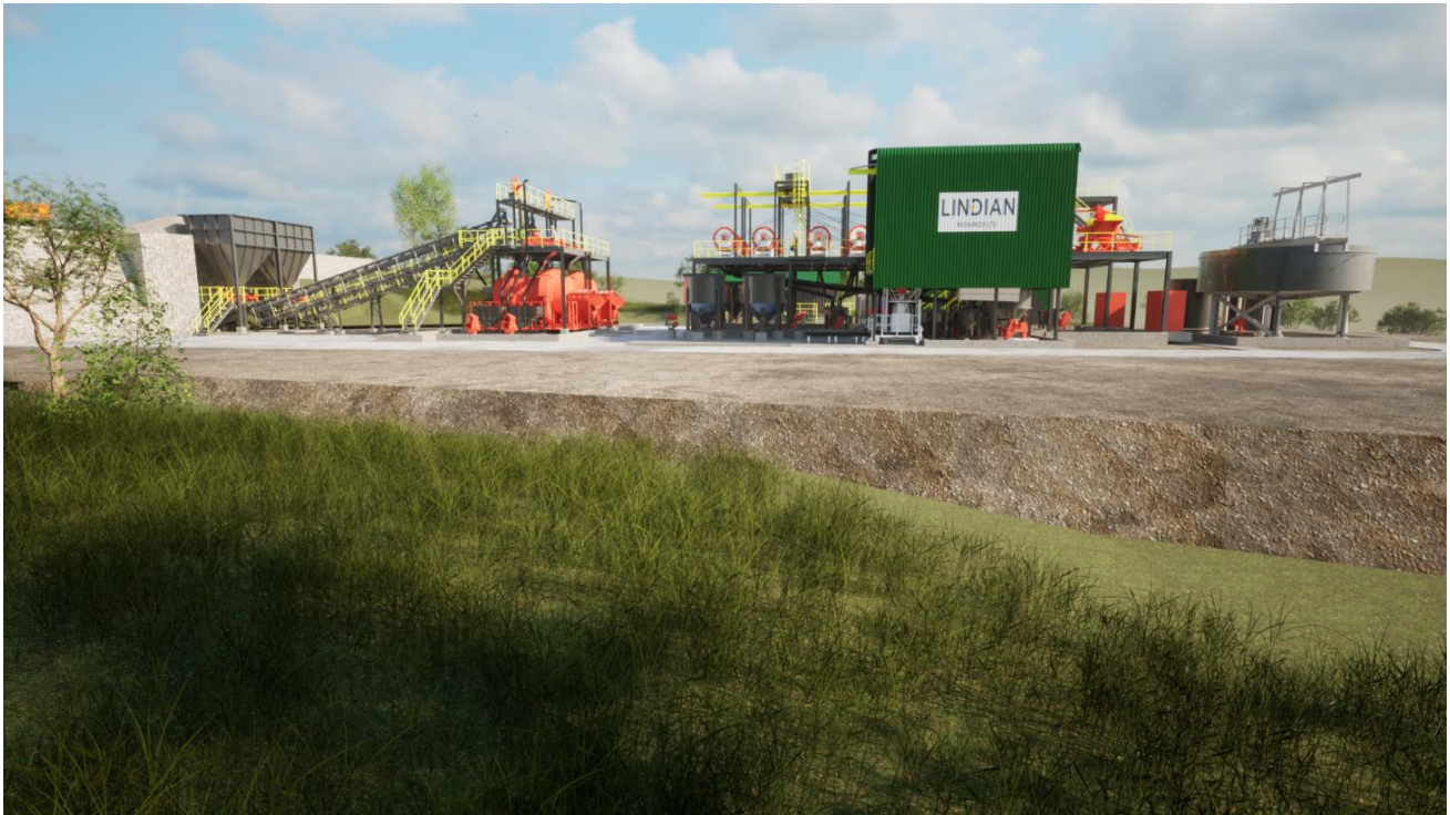
Image 1: Preliminary schematic of plant design from ground level. Existing retaining wall (left), ball mills (centre left), recovery circuit (centre) and tailings thickener (right)
