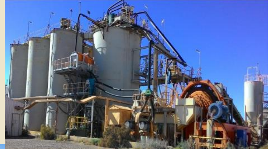
Processing Plant & Infrastructure in Laverton
