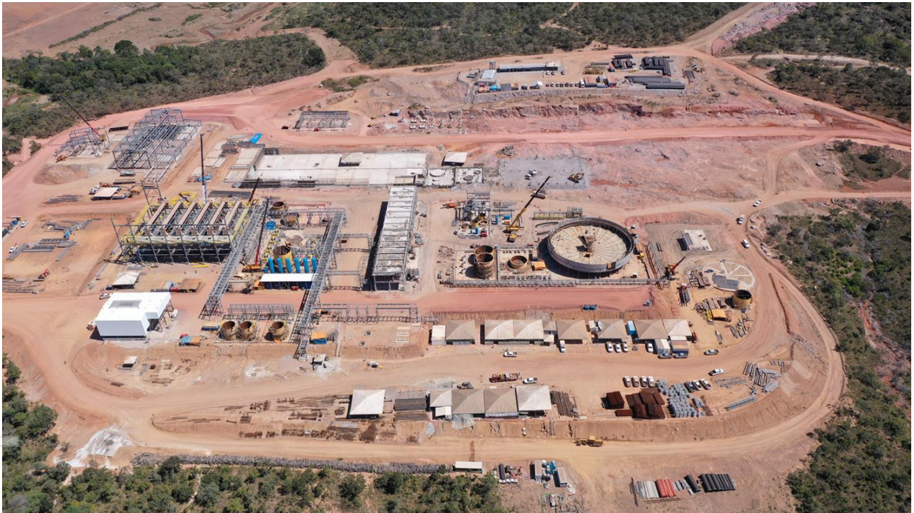
Figure 6: Serra Verde plant construction (taken in May 2022).
