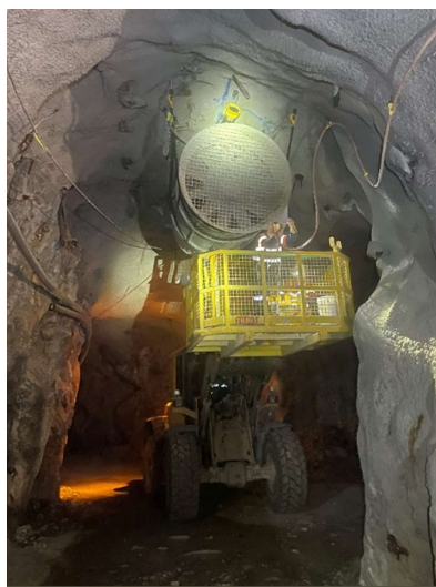
Figure 1: Underground portal, secondary ventilation fan installation and pumping at Mineral Hill underground.
