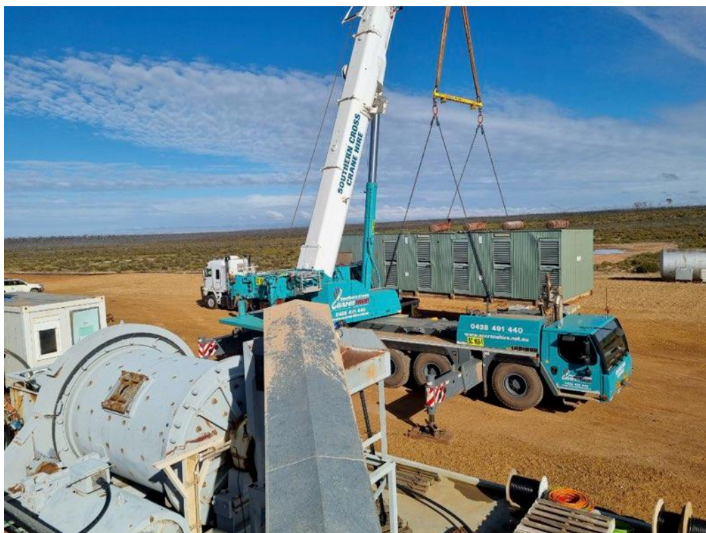
Figures 4 & 5: Crane lifting power plant and close-up of processing plant.
