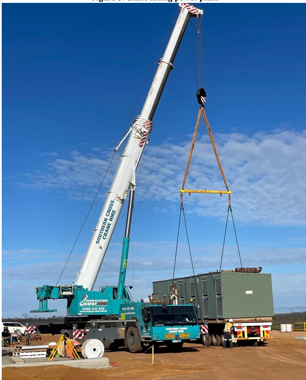
Figure 3: Crane lifting power plant
