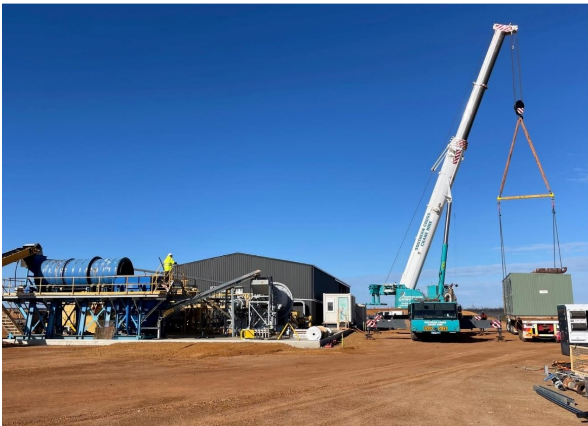
Figure 2: Crane lifting power plant
