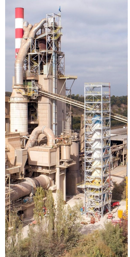
The ZESTY reactor will be the same scale as Leilac-1 reactor for cement and lime
