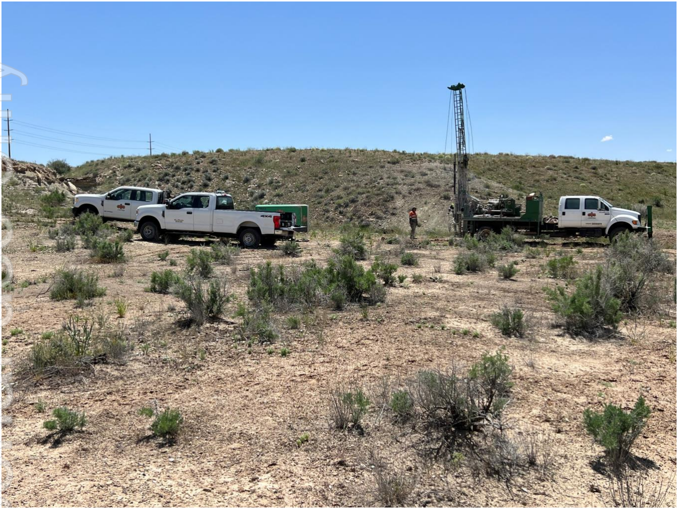
Figure 1: Photo showing the drilling rig on site carrying out geotechnical engineering work. Powerline infrastructure within the property is also shown.
