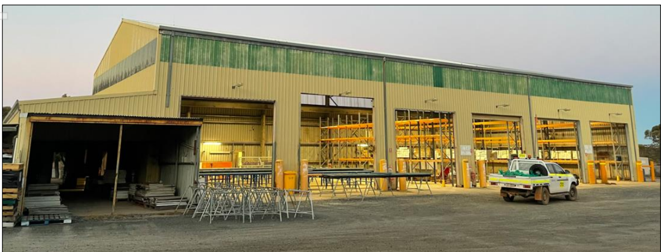
Figure 19: Foster Mine workshop
