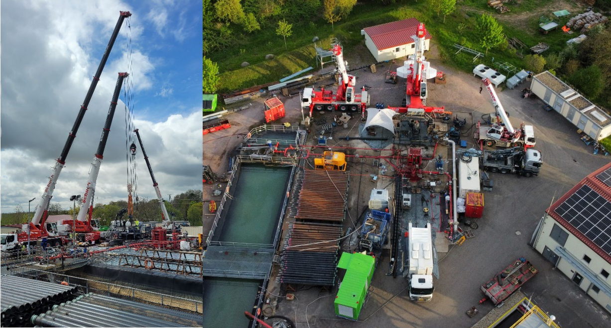
Cranes supporting Insheim pump change
