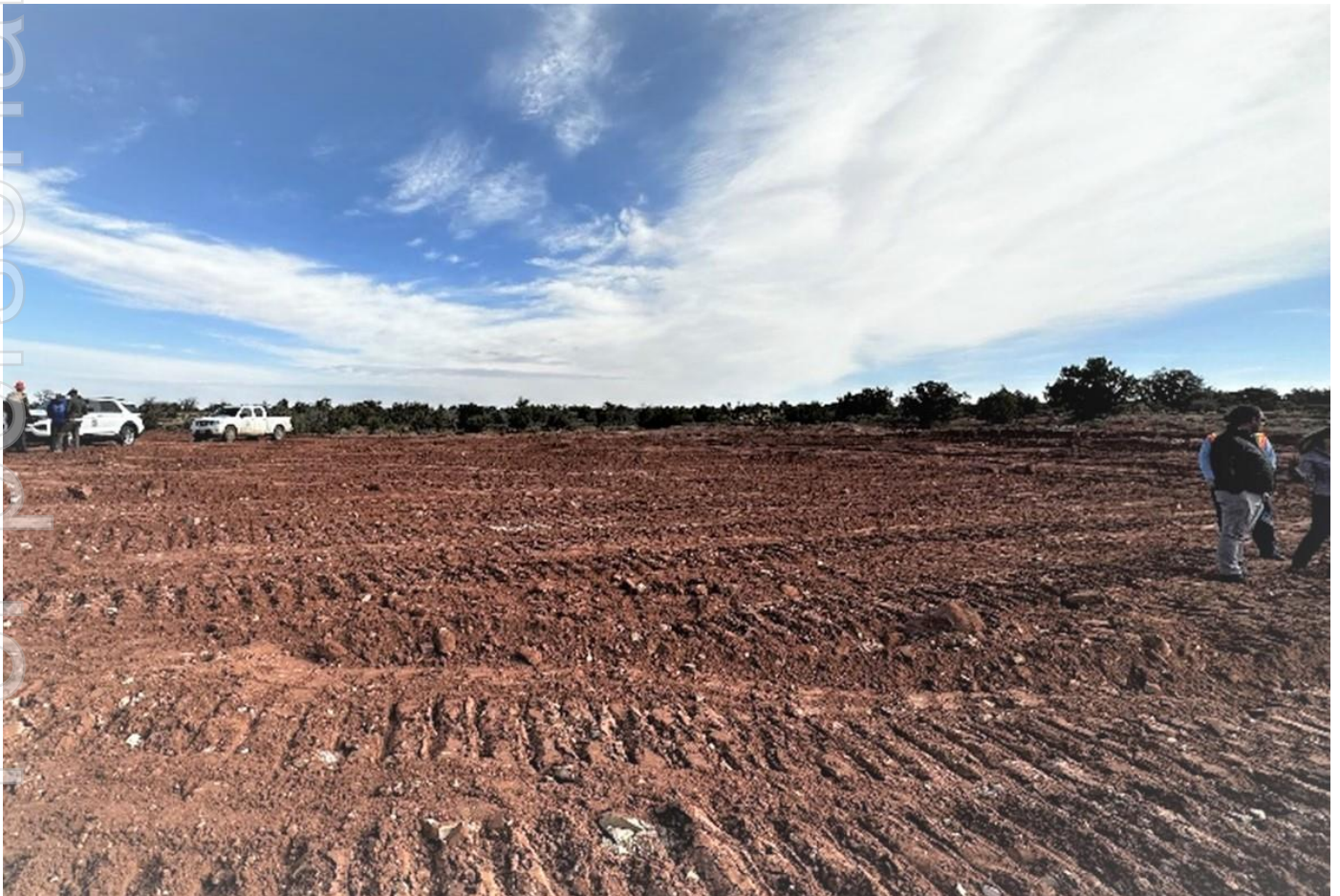
Figure 1: Federal and State personnel inspect the re-instatement works on the Mineral Canyon pad.
