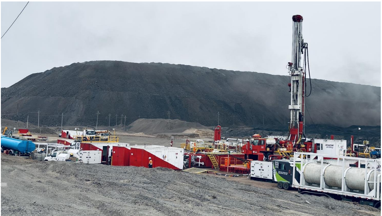
Figure 1 – Major Drilling Rig on location for the Lucky Fox - 2 pilot production well
