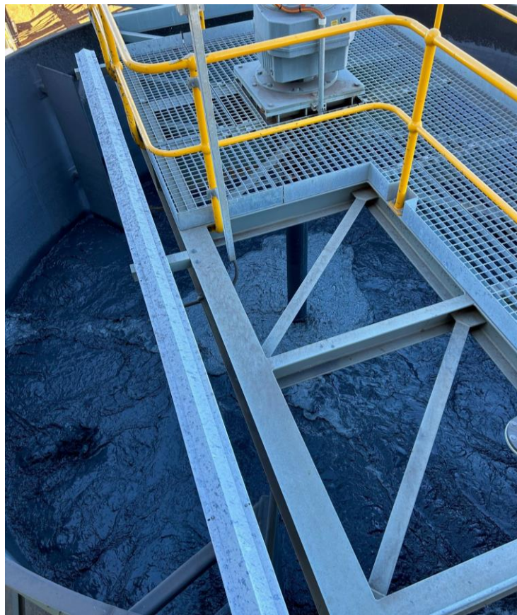
Figure 3 – Concentrate tank filling (photo 3 May)
