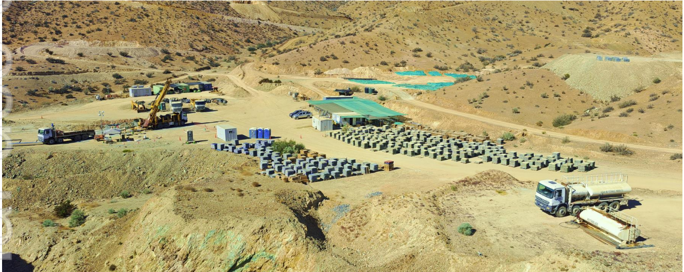
Drilling operations adjacent to the Cortadera core yard, Costa Fuego copper project, Chile, February 2023
