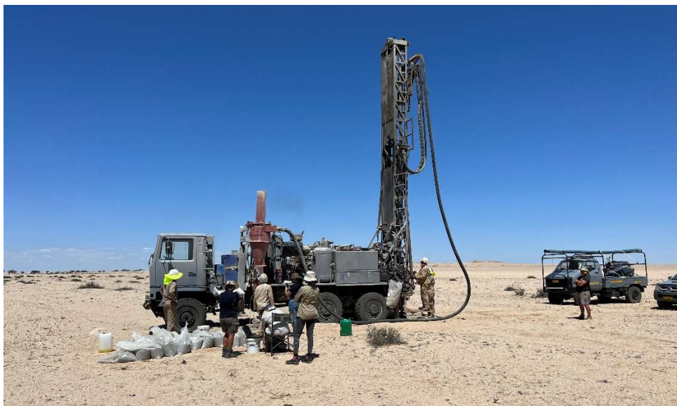
Figure 2 Drilling at Koppies 4
