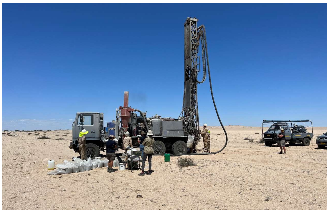
Figure 2 Drilling at Koppies 2 Extensions
