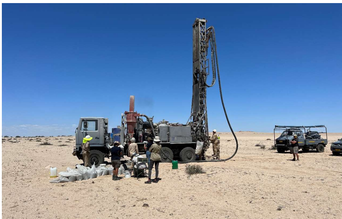
Figure 2 Drilling at Koppies 2 Extensions
