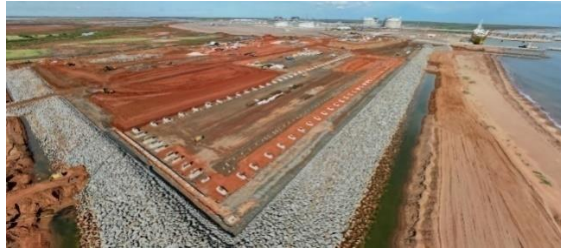
Product storage shed backfill at Port of Ashburton
