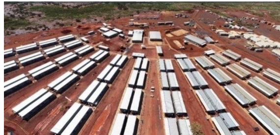
350-person construction camp at Ken's Bore
