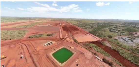
Runway apron and airport terminal bulk earthworks at Ken's Bore
