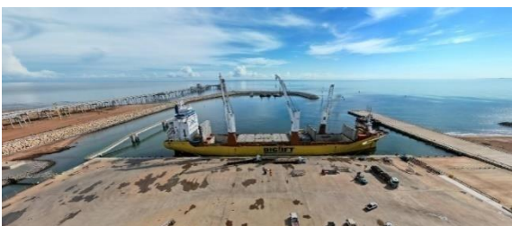
Big lift ship at Port of Ashburton unloading first steel shipment
