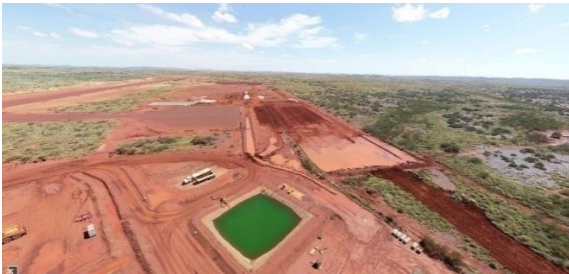
Runway apron and airport terminal bulk earthworks at Ken's Bore
