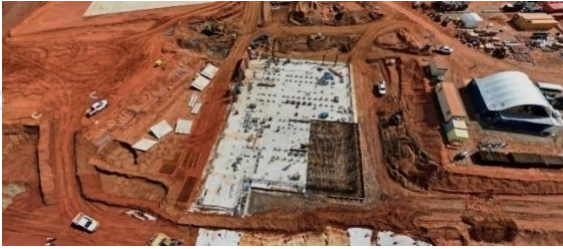
Unloading shed vault concrete progression at Port of Ashburton
