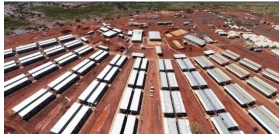
350-person construction camp at Ken's Bore
