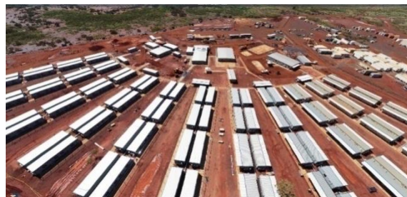
350-person construction camp at Ken’s Bore
