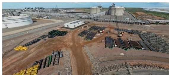
Cargo laydown from first shipment at Port of Ashburton
