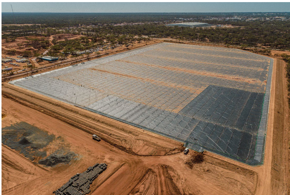
Kalgoorlie - Kieserite Evaporation Pond 3 – lining completed
