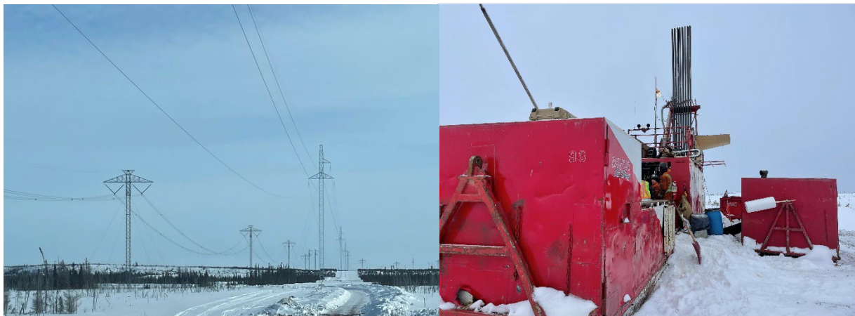
Figure 2: James Bay - Hydro-Quebec successfully installed powerline (left) and resource drilling (right)
