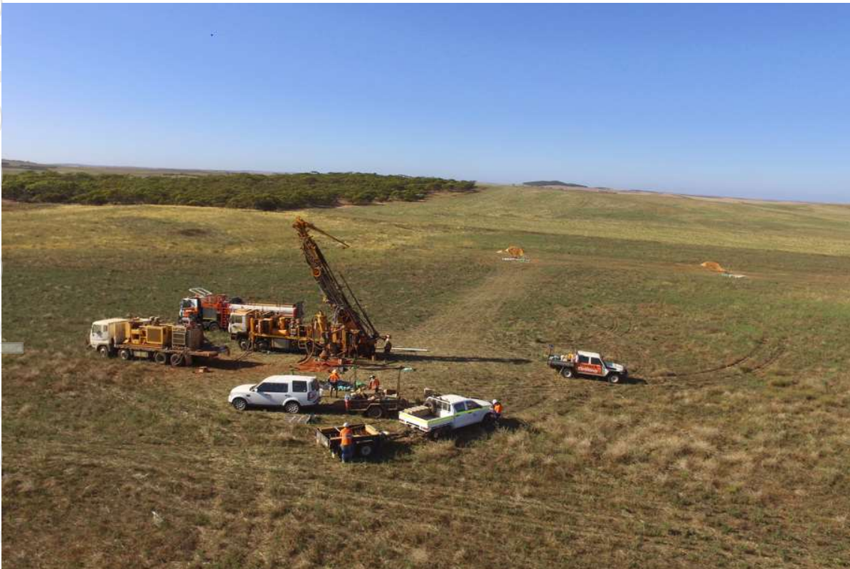
Figure 1: RC drill rig on location at Jamieson Tank in South Australia
