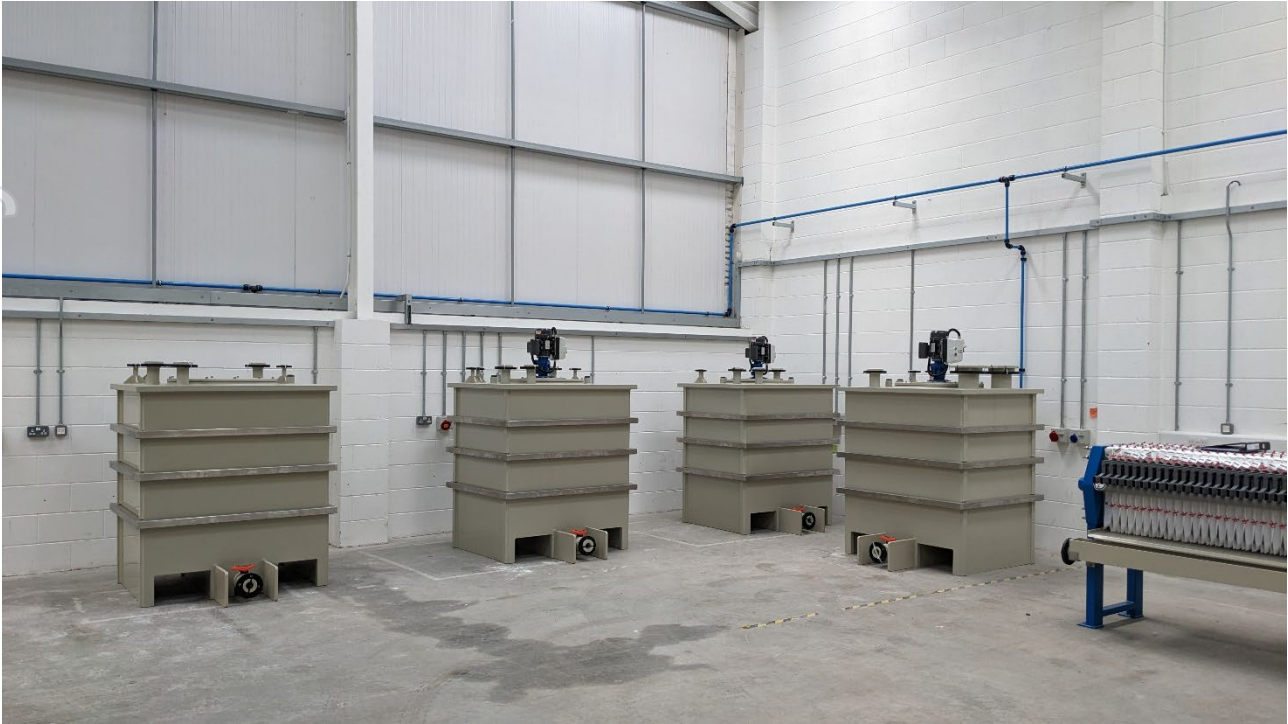
Figure 2: Process Reactors in position adjacent to installed utilities and services.
