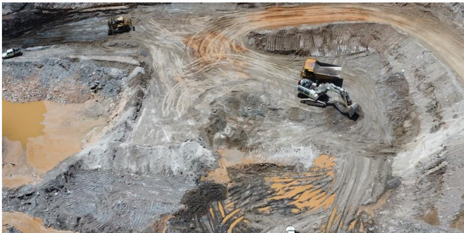
Dewatering of the Grants Pit was safely completed, and water management across Finniss is under control allowing for full mining operations to recommence in late March 2023.
