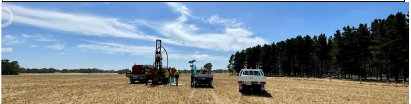
Drilling – Dovetail Region
