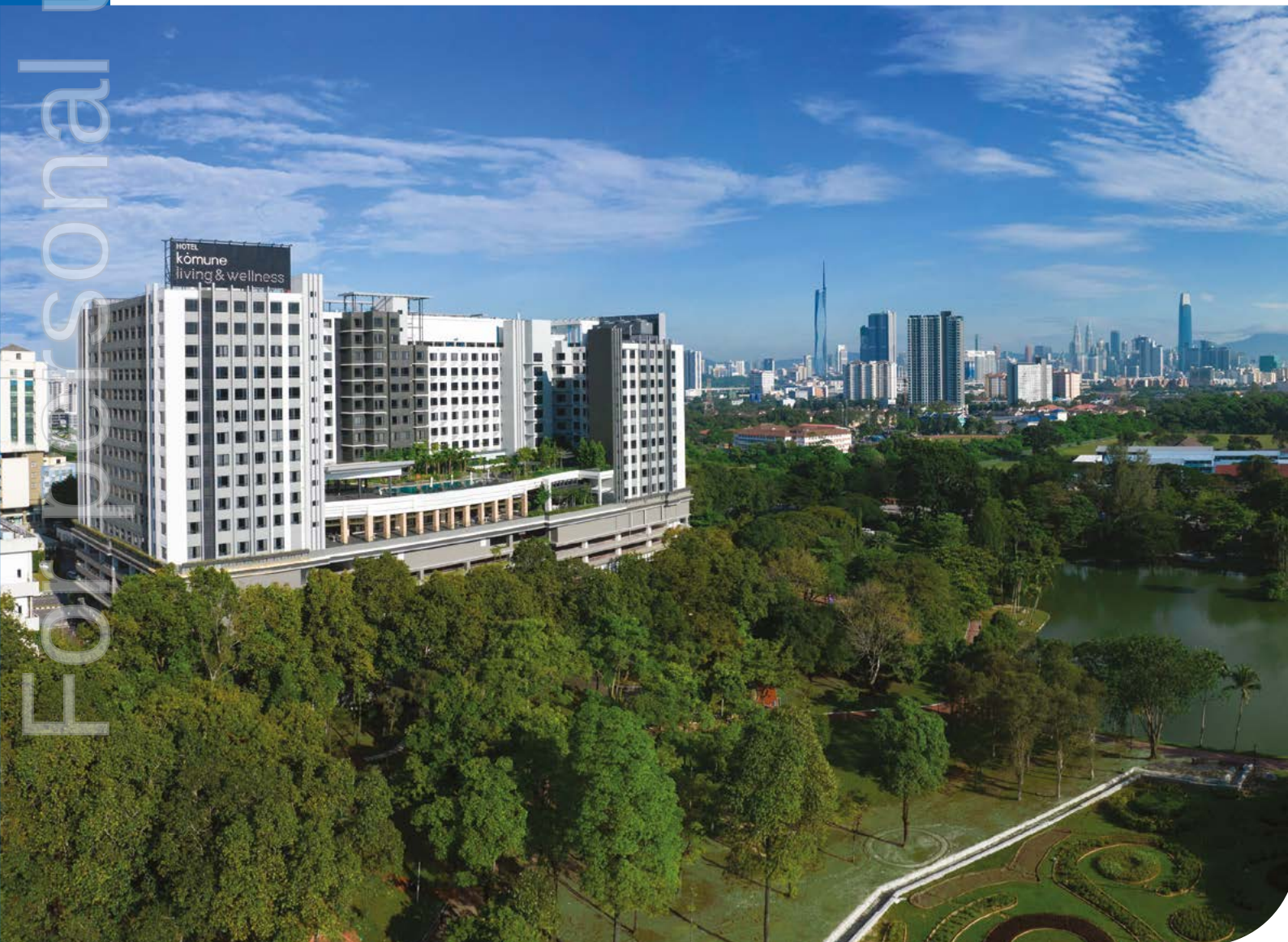
Komune Living & Wellness - Facade Park View
