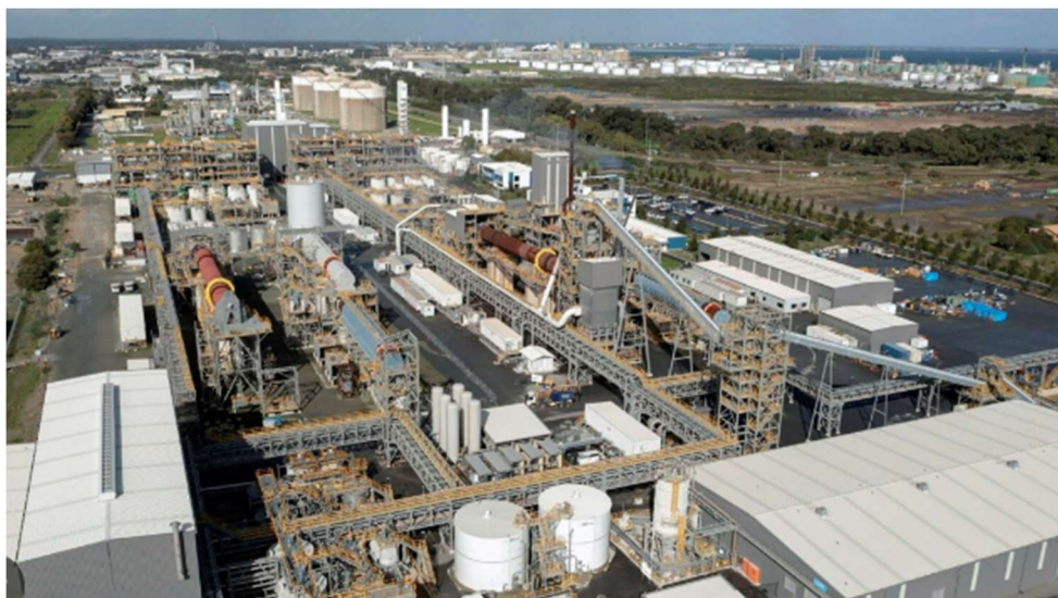
Figure 11 – Kwinana lithium hydroxide refinery
