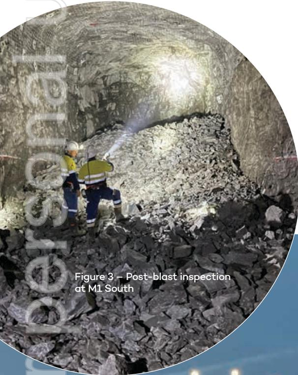
Figure 3 – Post-blast inspection at M1 South
