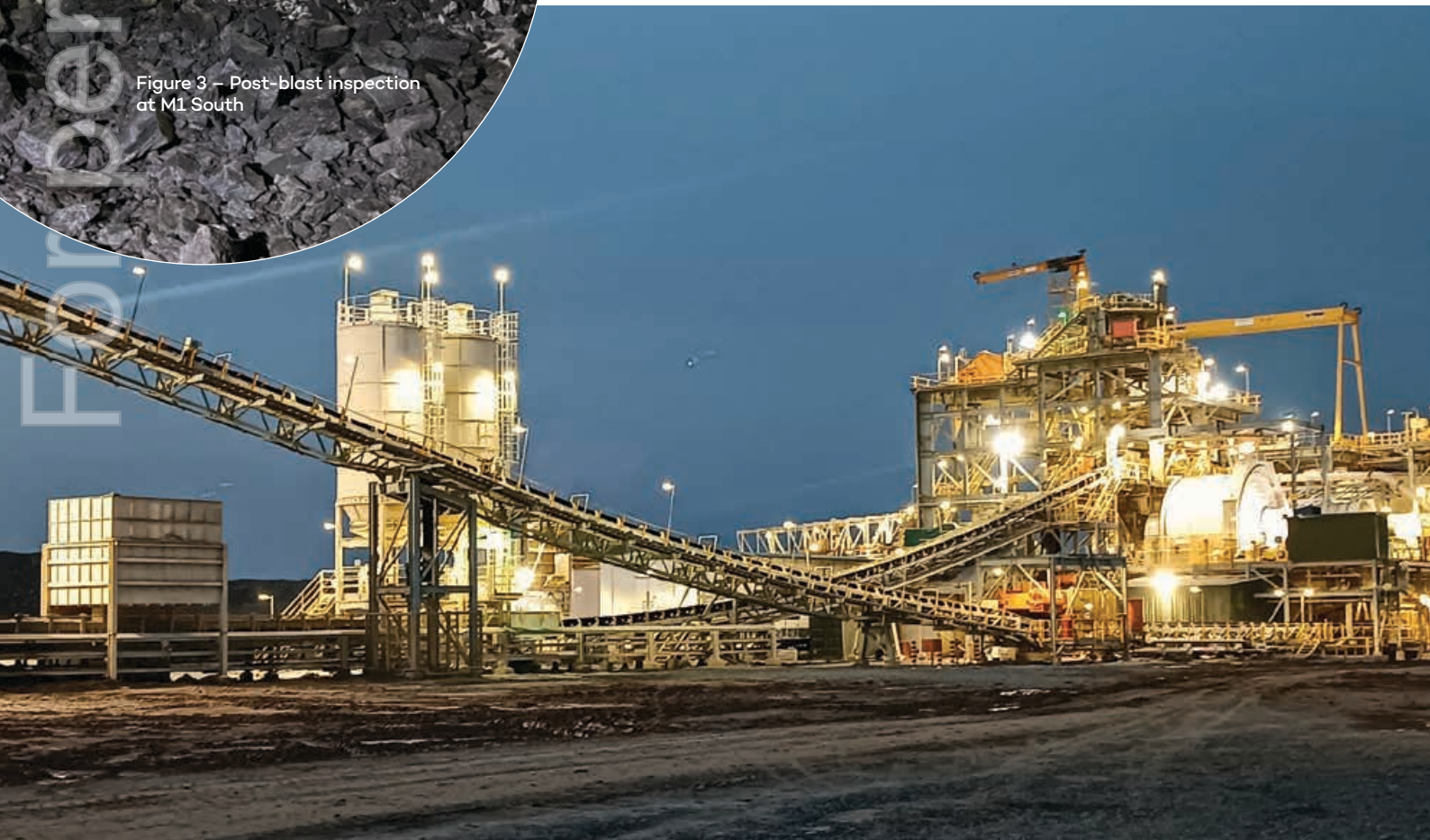
Figure 4 – Sanbrado process plant
