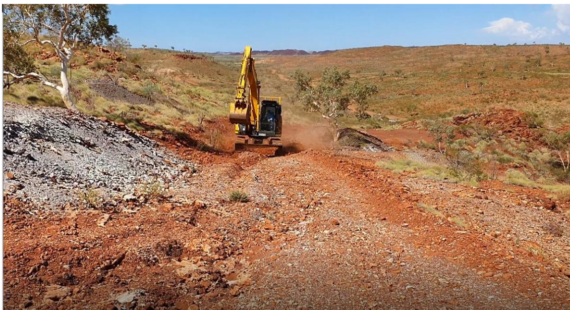
Figure 5. Repairing access track at Yannery
