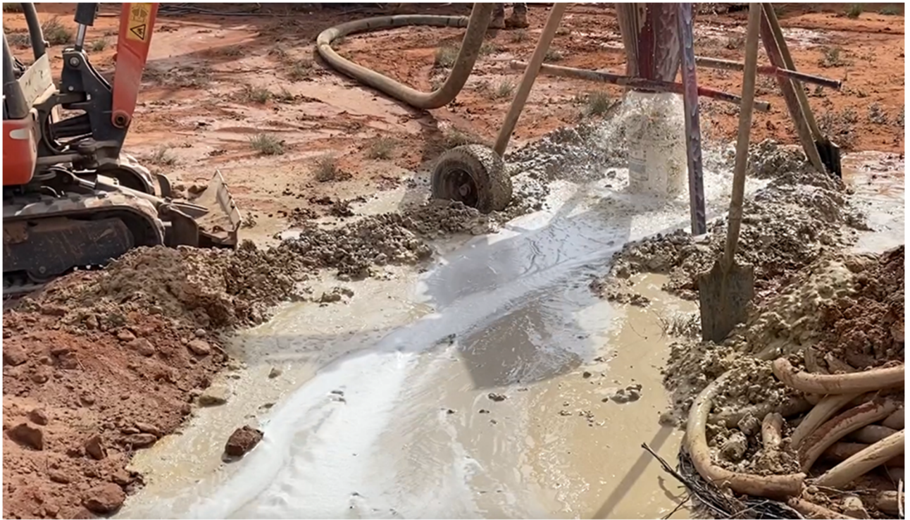
Figure 12. Brine flowing from cyclone at 78m from LWP002.
