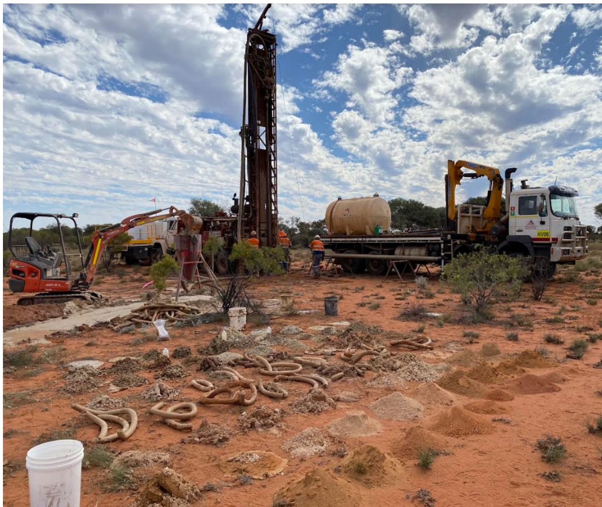
Figure 11. Water Well rig drilling at LWP002.
