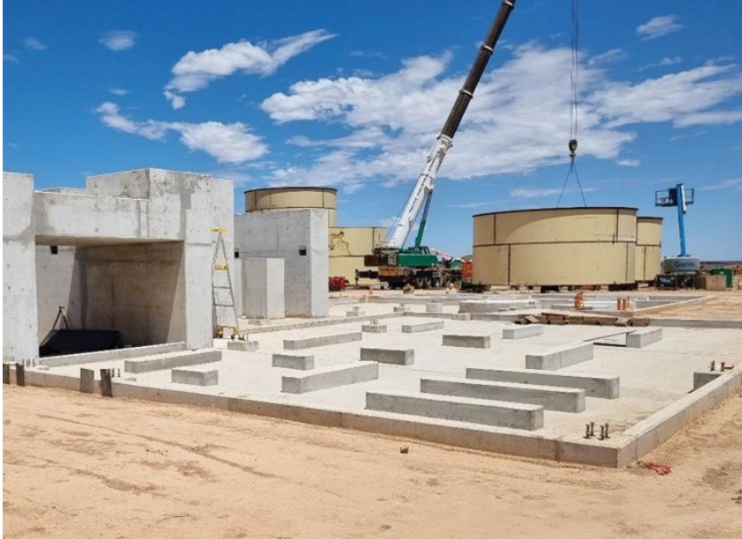
Figure 6: Construction progress on the ball mill foundations at the processing plant as at 24 January 2023
