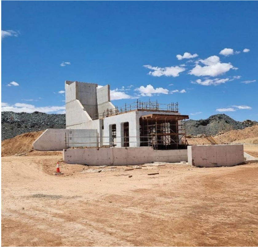
Figure 5: Construction progress on the Primary Crusher facility at the processing plant as at 24 January 2023
