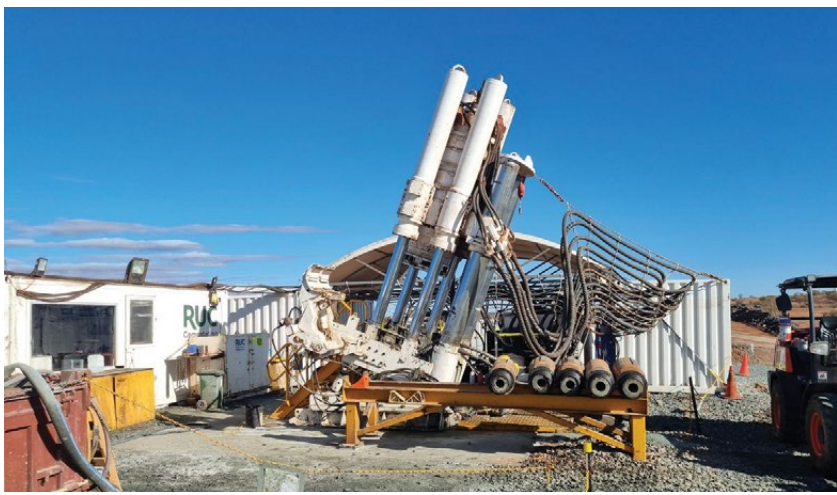
Figure 8: Bellevue site RUC raisebore drilling at the Northern escapeway rise (right); Second raisebore drilling rig at the Southern ventilation rise (below right)
