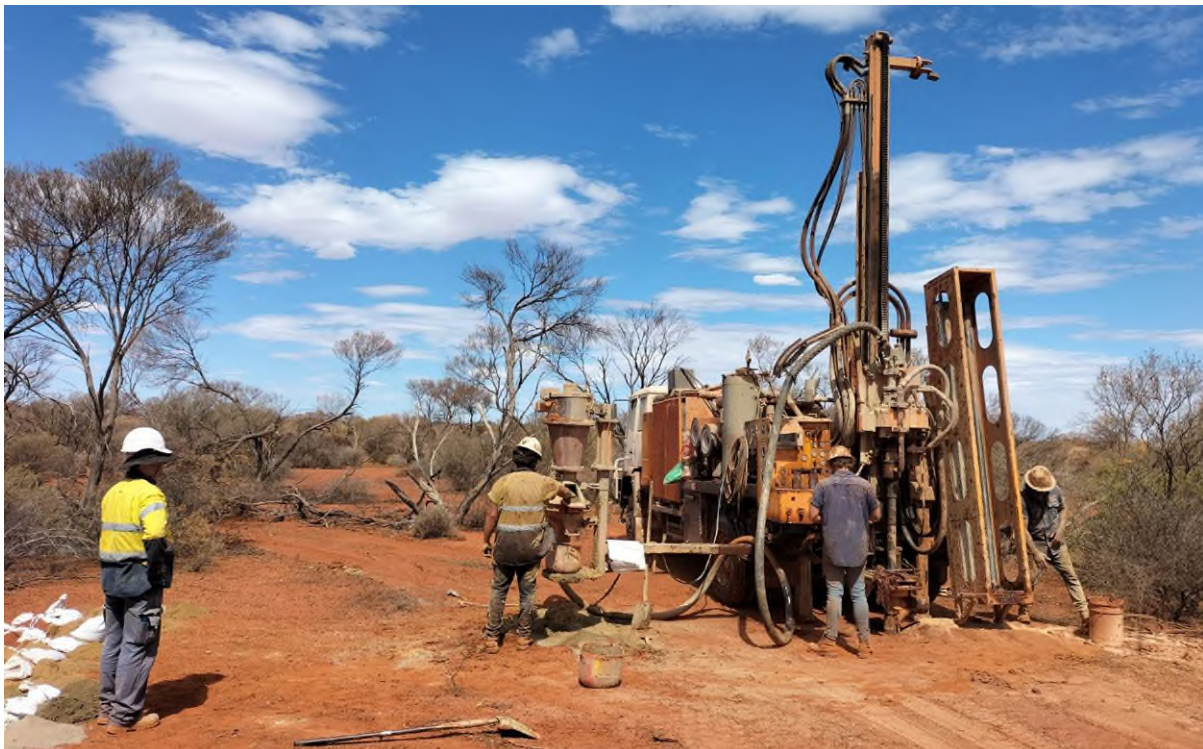
Figure 1: Aircore drilling underway at the Pt Kidman Prospect in January 2023.
