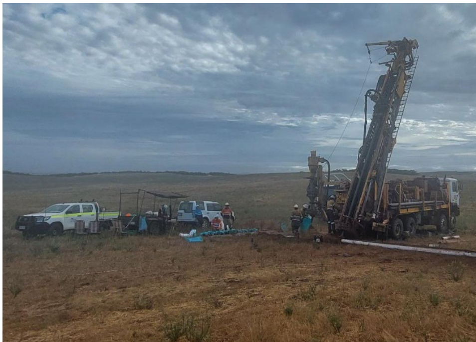
RCP drill rig on location – EL6634
