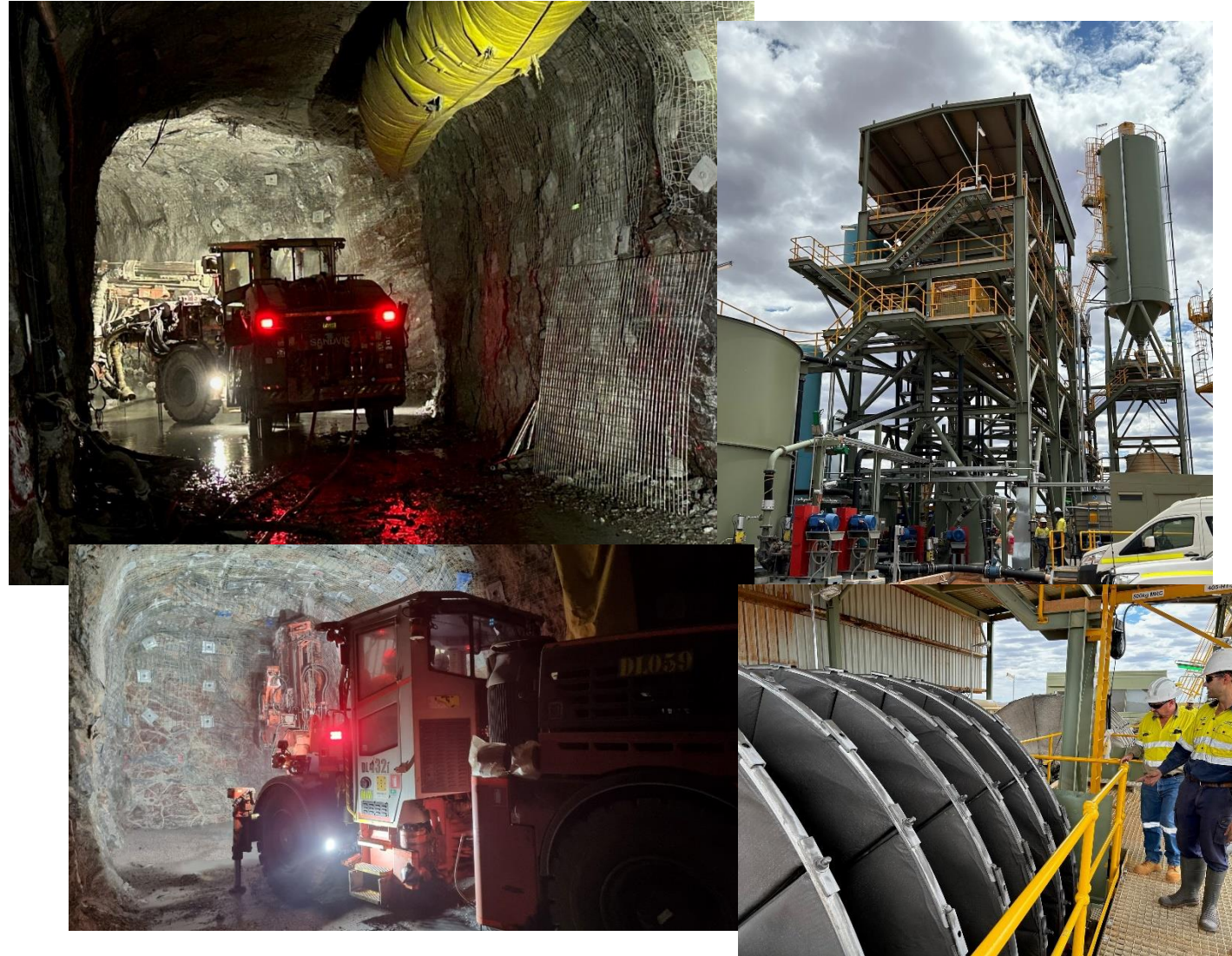
Figure 11, 12, 13 & 14: Abra underground development, stope drilling and paste plant
