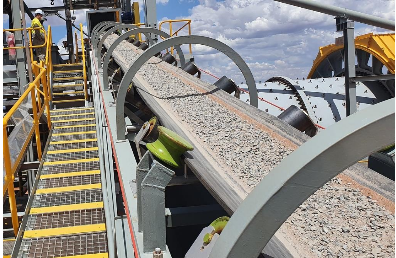
Figure 4: First ore being fed into mill at Abra (Photo dated 9 January 2023)
