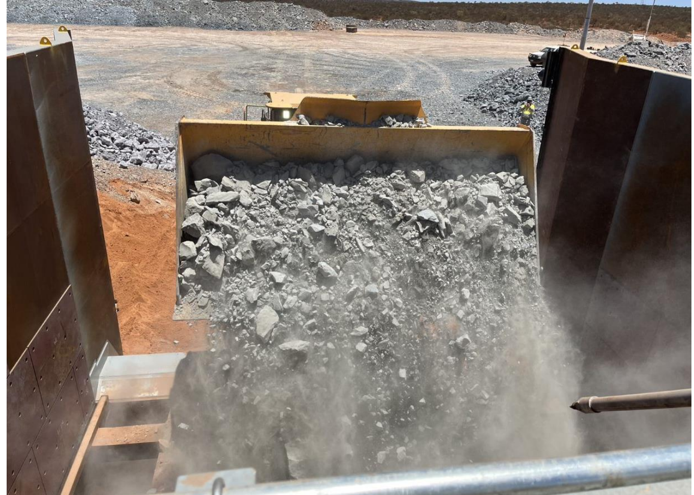
Figure 3: First material being tipped into crusher during commissioning (Photo 26 November)
