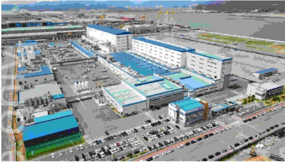
POSCO cathode material plant in Gwangyang, South Korea
