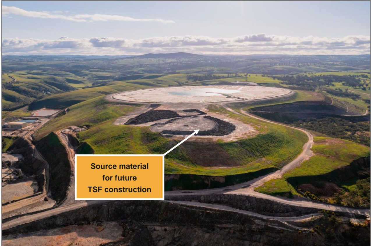
Figure 48: Integrated waste landform showing rehabilitated areas and open areas containing waste rock for future TSF construction
