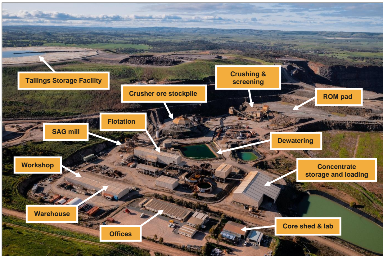
Figure 40: Kanmantoo Copper Mine processing plant and workshops
