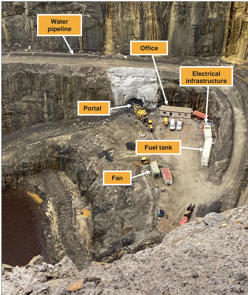
Figure 52: Infrastructure located at the underground portal
