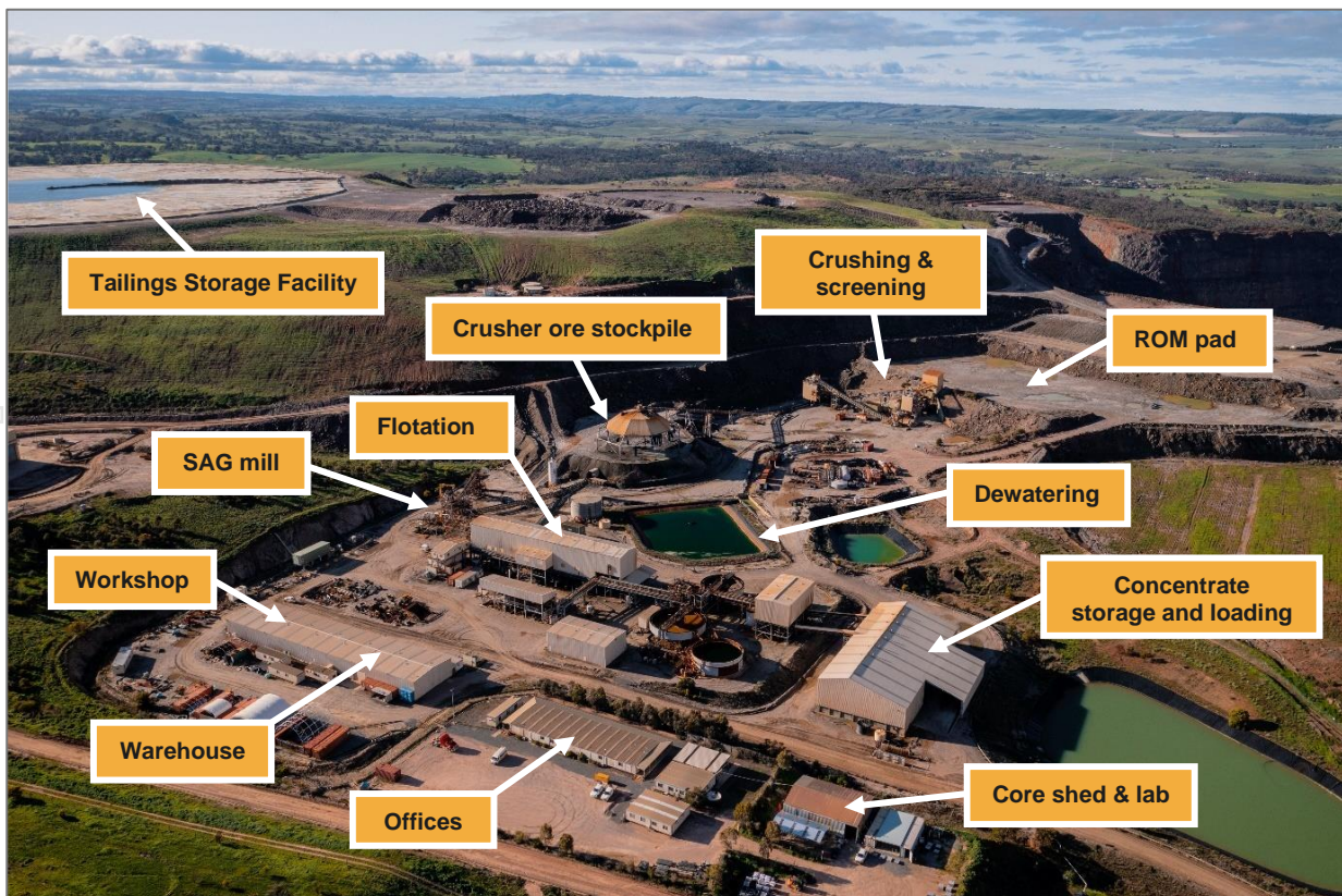
Figure 40: Kanmantoo Copper Mine processing plant and workshops
