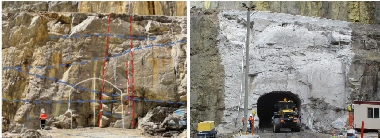
Figure 24: Mapping of the dominant geotechnical features in the exploration decline portal face (left) and the established 900 exploration decline portal (right)
