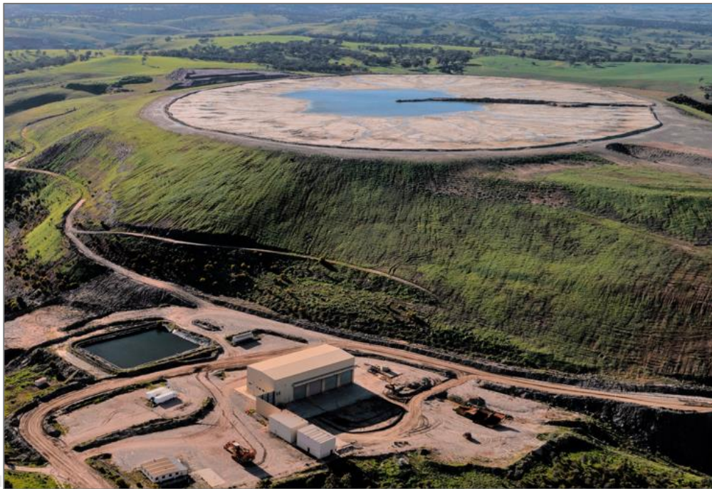
Figure 54: South facing photographs of the IWL in January 2020 (top) and August 2021 (bottom) showing rehabilitation revegetation and landform shaping
