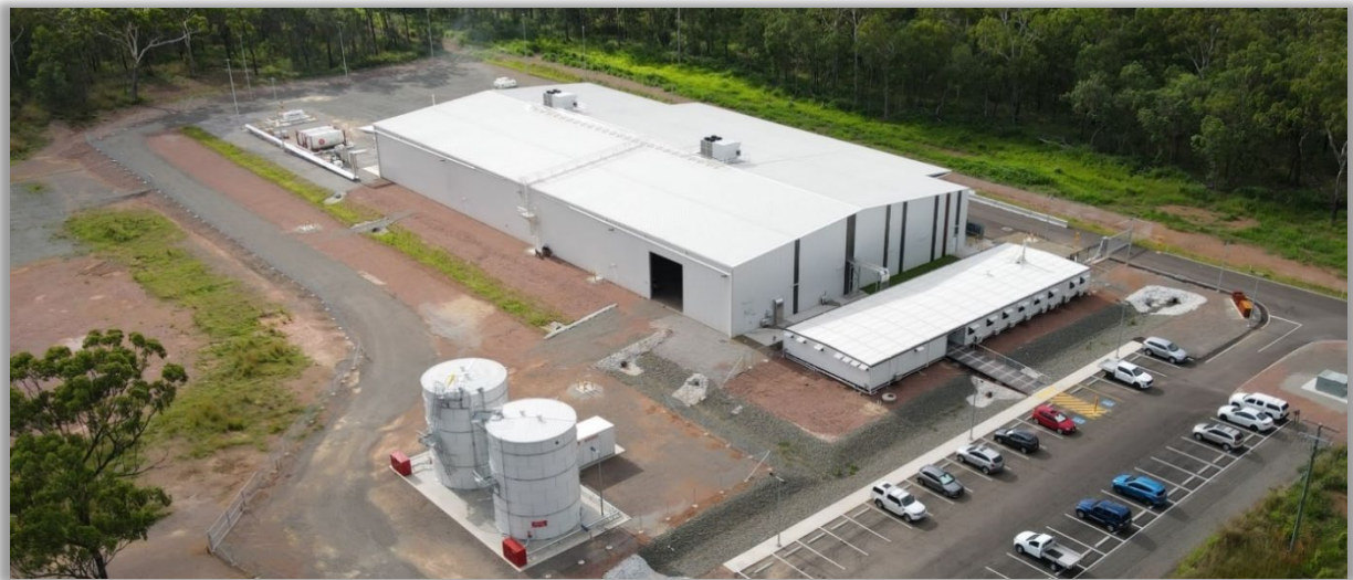
Completed Stage 1 PPF
