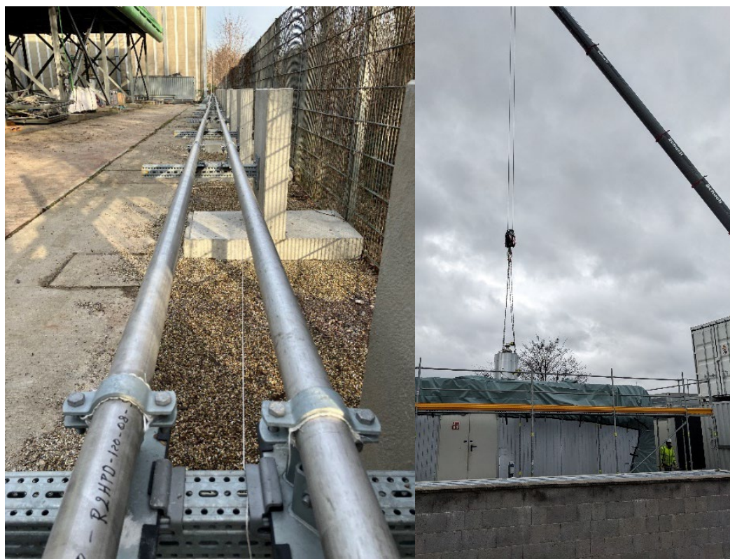
Figure 1: Brine line installation and construction progress at Vulcan's Lithium Extraction Demonstration Plant at Landau
