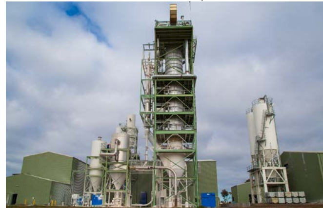
Electric kiln using flash calcination technology developed by Calix
