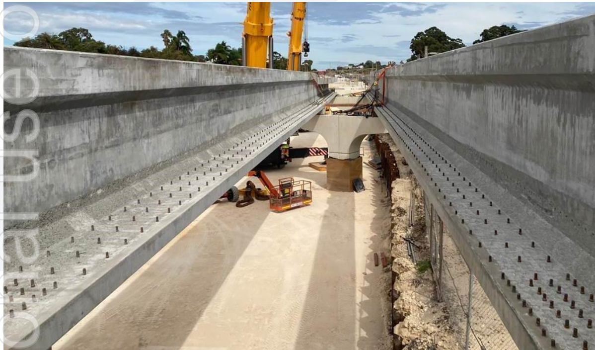
Beam Installations at Bayswater Train Station
