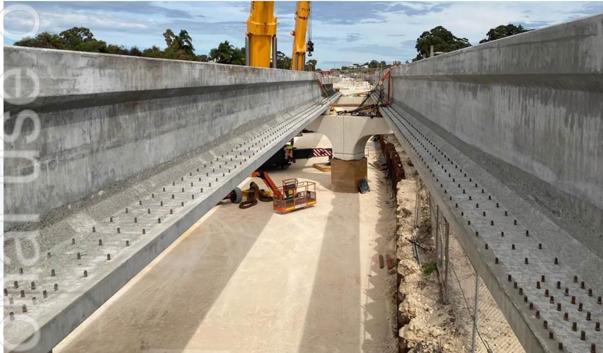
Beam Installations at Bayswater Train Station
