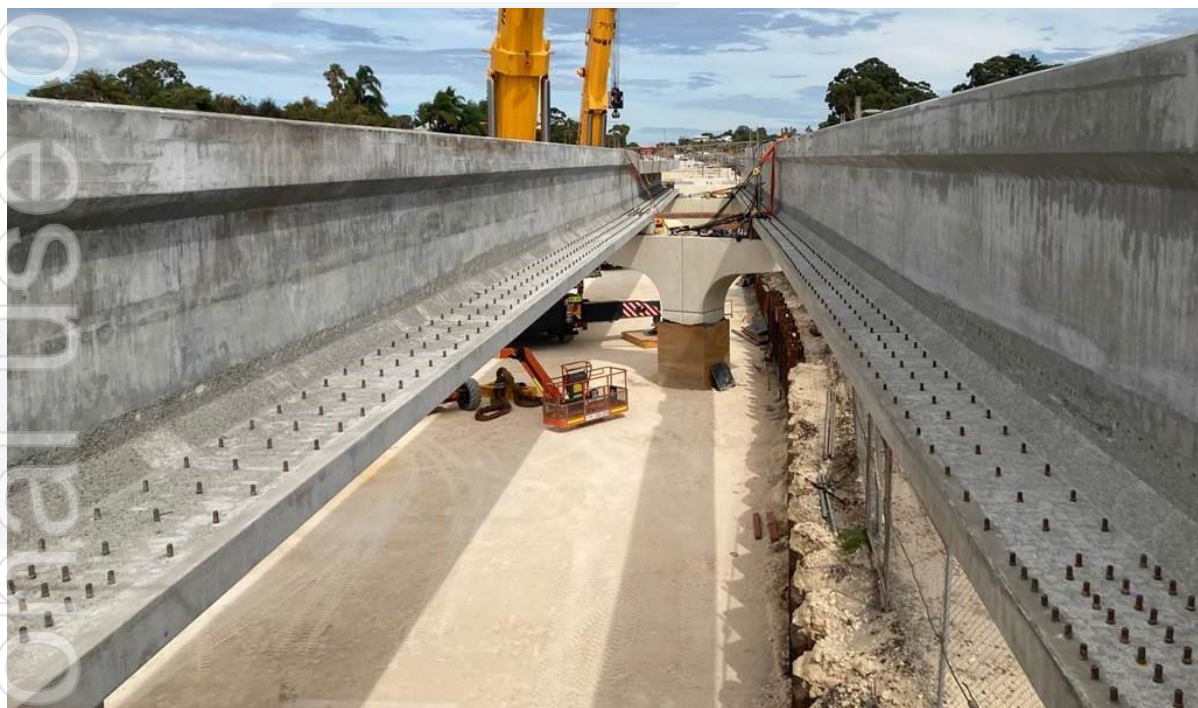
Beam Installations at Bayswater Train Station
