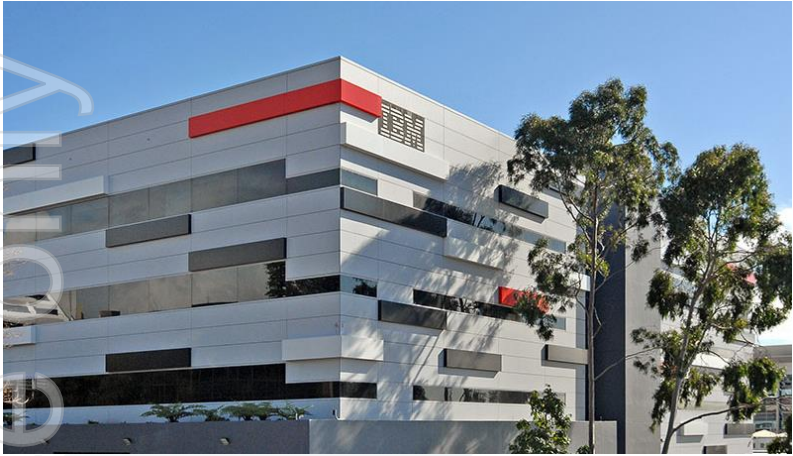
Fugro Building West Perth, WA
