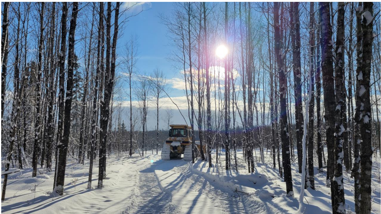
Photo 1: Dozer preparing access tracks and drill pads - 2021/22 Drilling Campaign
