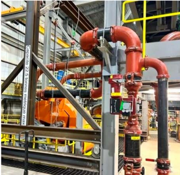
WHIMS rubber-lined piping installation (left); gate valves (right)
