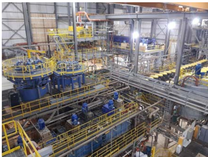
New WHIMS (left) and desliming sector (right)
