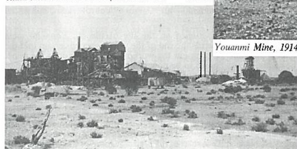
Weathering structures, Youanmi Gold Mine, 1933 (A.E. Lefroy)
