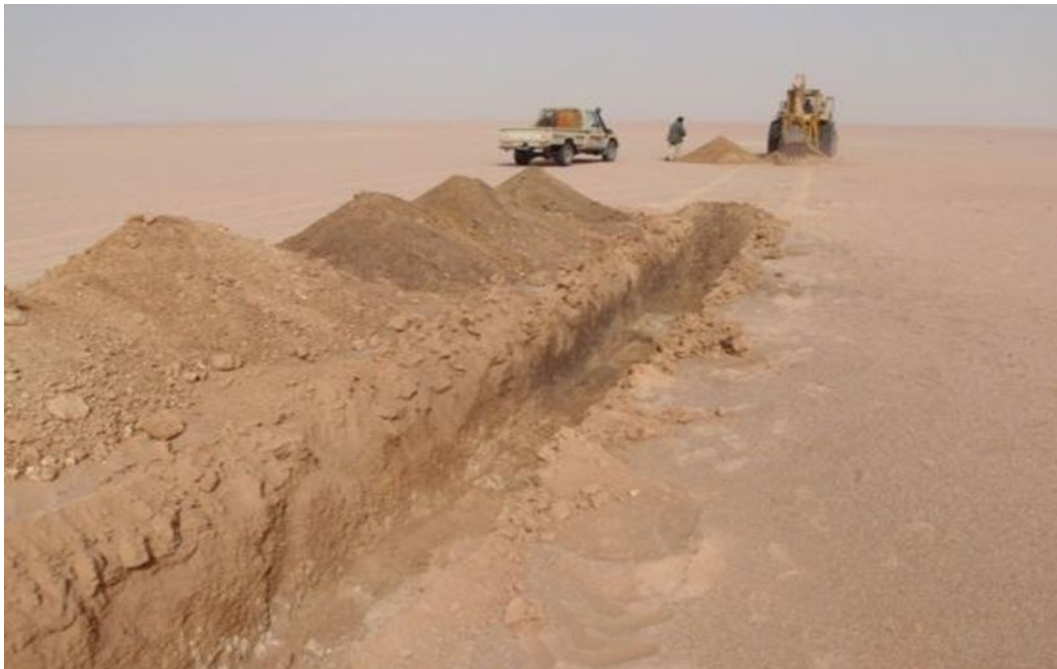
Figure 4: Typical landscape within Tiris Project area, trench illustrating soft sandy overburden with gravelly calcrete beneath
